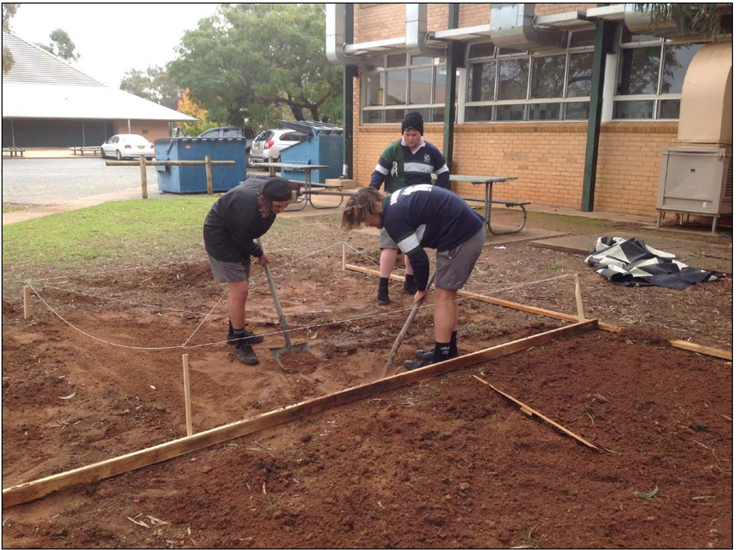
Above: Some of the work studies students building the games area.
